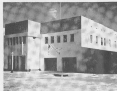
Douglas City Hall remodeled in 1951
